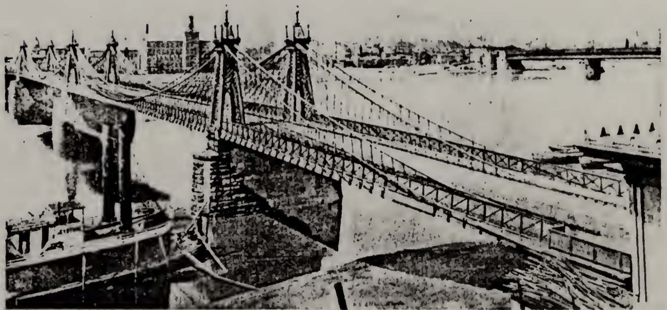
The Pittsburgh-Allegheny Bridge, Completed in 1860
